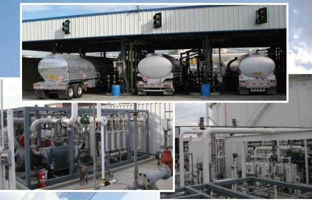
The ARID Membrane CRU (Carbon Retrofit Unit) Gasoline Vapor Recovery System is installed at high capacity, bulk terminals for reducing hydrocarbon emissions while at the same time increasing loading rack rates.
